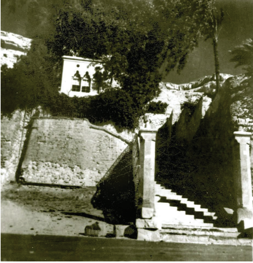
(Pl. 4) The main staircase leading to the main entrance of the convent ( https://www.facebook.com/photo/?fbid=10151636565178290&set=a.10151336424388290 )
